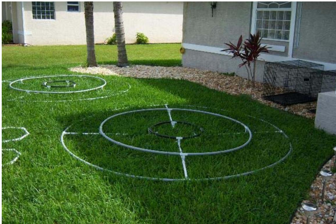
**15. Now take (2) of the 3/4" Gray Electrical PVC Conduit and make you interior LIGHT RING. Take your extra (4) Double Tees from step 11 and attach the light ring to the 45" horizontal supports.**
