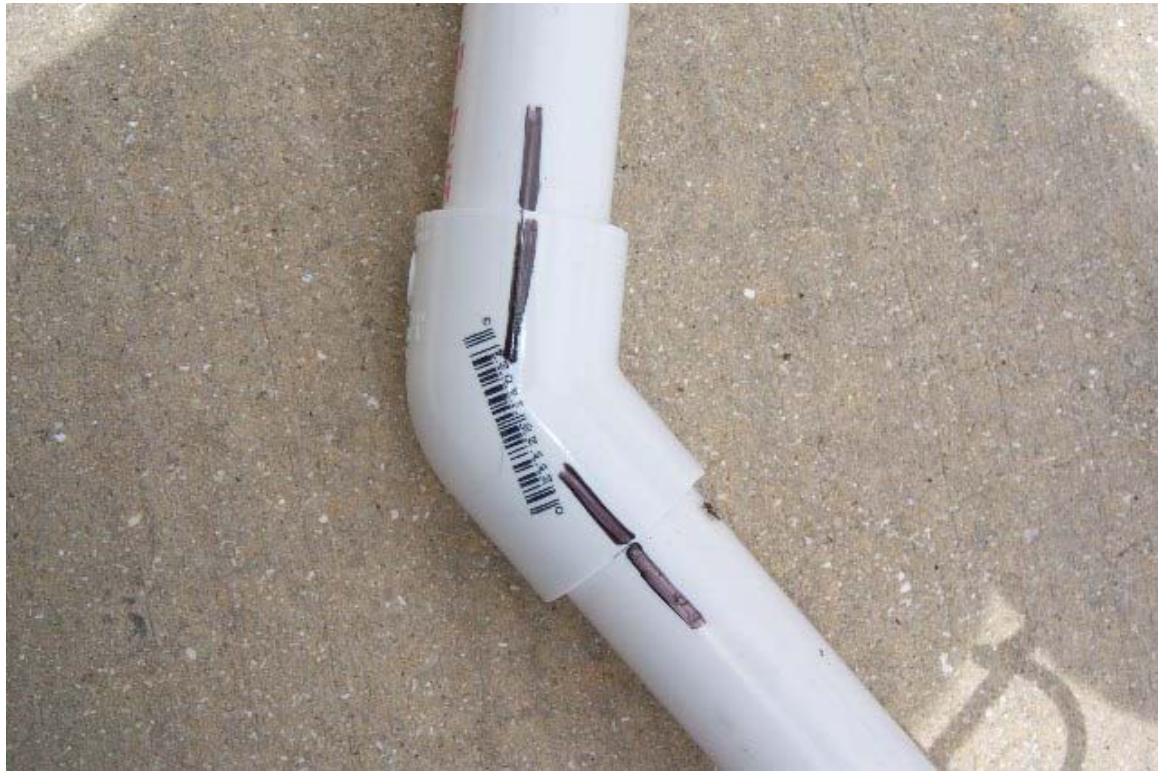
**6. Using a "Sharpie" or similar, and with the octagon lying flat, make a series of lines on both the elbow and the PVC pipe where it inserts into the elbow. Now when you glue it together, do one connection at a time and work your way around the octagon without skipping. Even if it moves a little you still know where it has to be just by LINING UP THE MARKS YOU MADE. This is the easiest way I have found to make sure it is flat and straight.**
