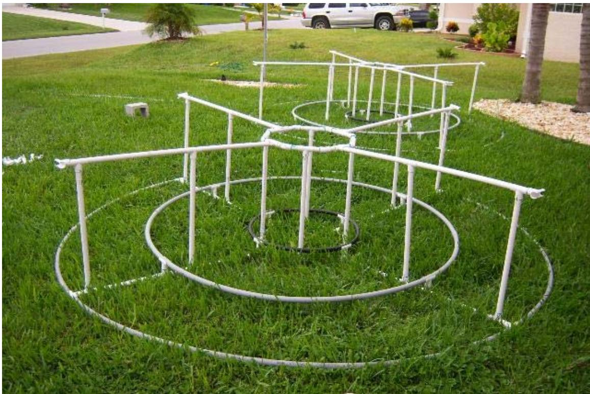
**22. Now add the last (4) vertical supports near the center of the horizontal supports.**
